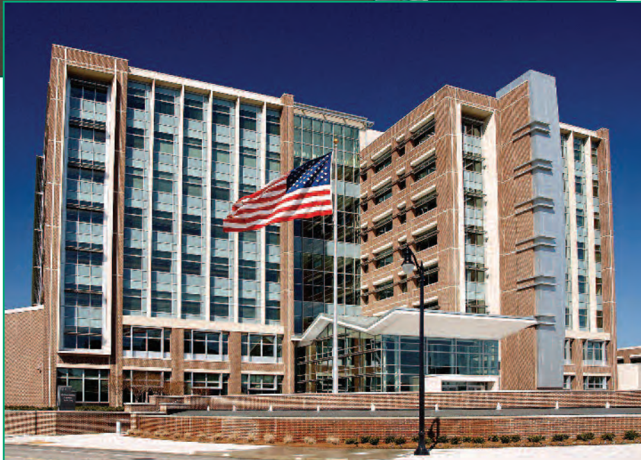
Top: Before installing the overburden, Construction Services loose-laid a polypropylene composite with a drainage core and a water-retention fabric on one side on the waterproofed deck. Bottom: The completed Birmingham Social Security Administration Center has achieved LEED® Silver Certification.
